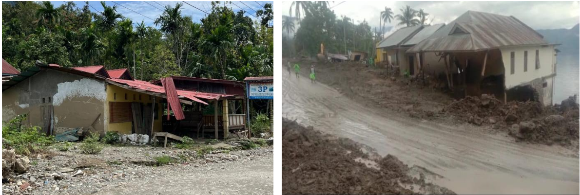
Figure 3. Condition of Residents' Houses Damaged by the Galodo Flood in Jorong Tanjung Sawah (Source: Community Documentation, 2025)
