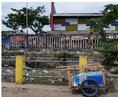
Figure 8. The Market Fence That Separates the River From the Market Area Source: Author Documentation (2022)
