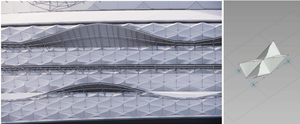
Gambar 5. Dinding fasad material *plastic composite panel fabrication*
